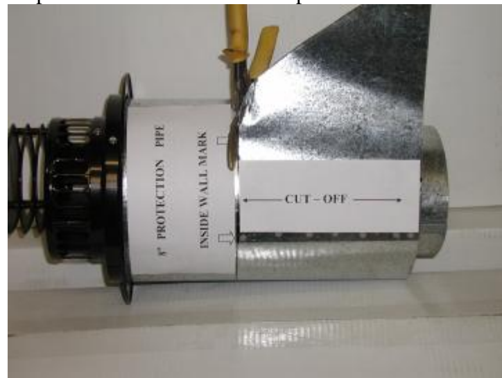
Step 4 – Cut off 8” Protection Pipe excess at wall mark.
