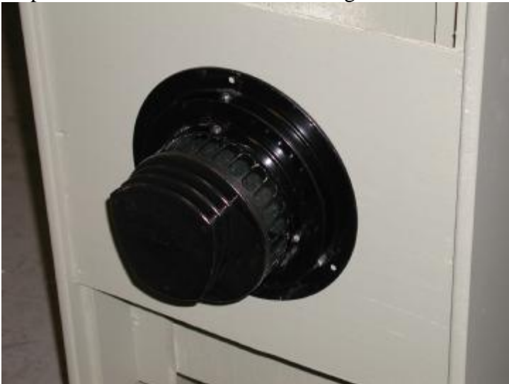
Step 2 – Place vent in hole for marking.
